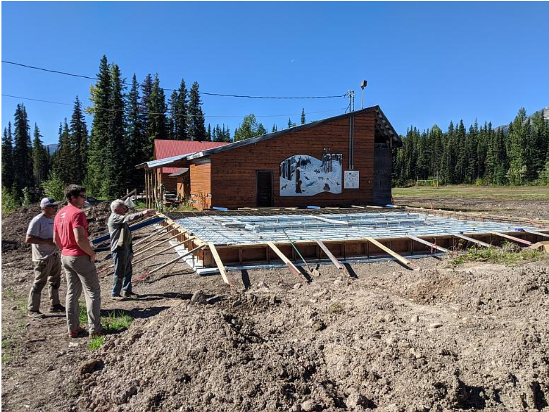
Tracksetter garage foundation under construction, September 2020
