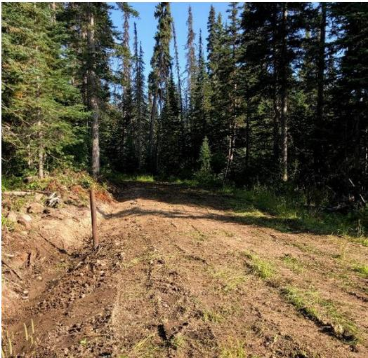
New subgrade at wet spot on Hound Heaven near Jct I. Tractor would get stuck here and wet ground prevented early season skiing.
